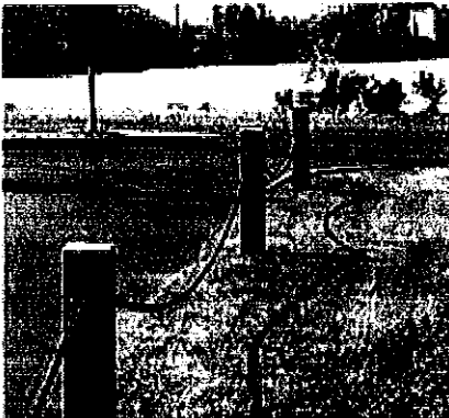
Granite Posts. 6" x 6" granite posts with black powder coated chain. 10' apart spacing
