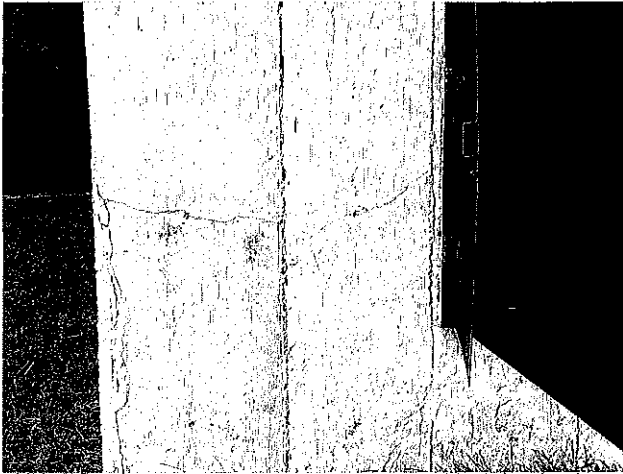
11 – Horizontal and vertical crack at south end of the east side similar to those at the north end.
