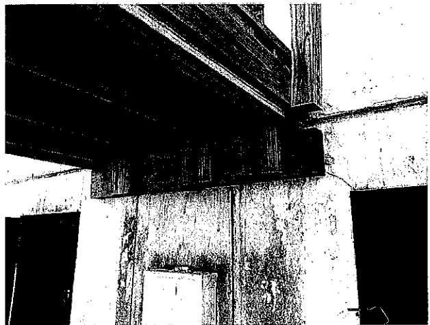
21 – Connection of ledger to concrete wall appears to be inadequate.
