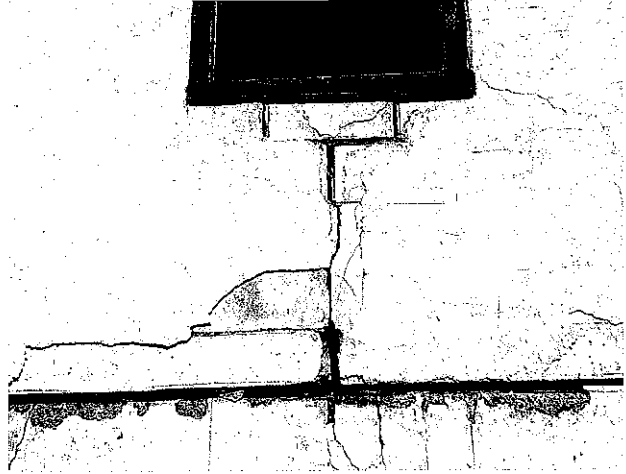
14 – Large open mortar joints in the concrete block in the middle of the south wall.
