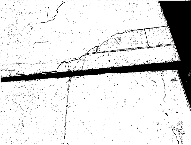
12 – South side. 2 nd floor slab does not align with concrete wall below.
