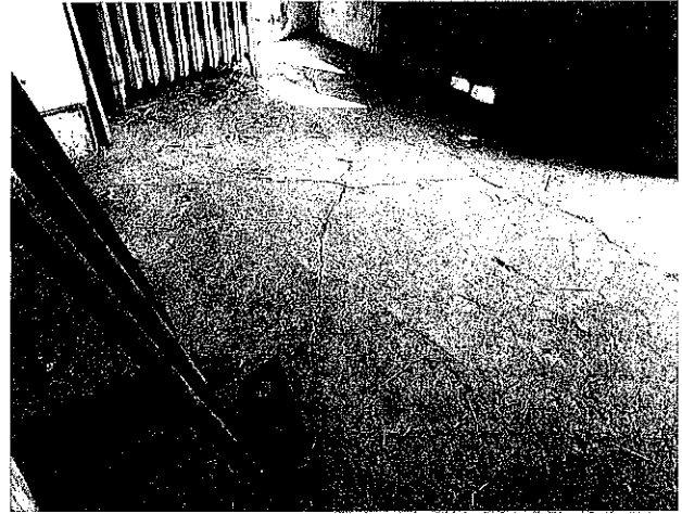
31 – 1 st floor, northeast room. Cracking of slab-on-grade.
