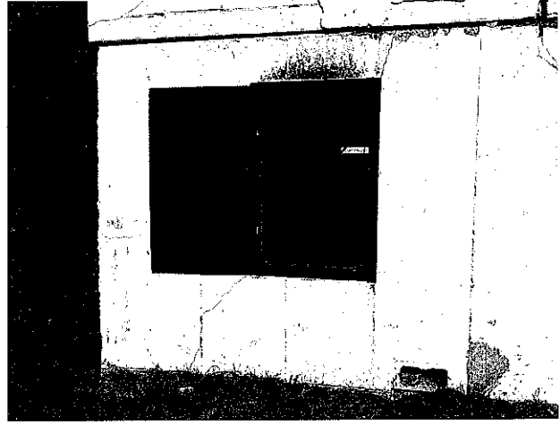
15 – Horizontal and diagonal cracks at west window on south side.
